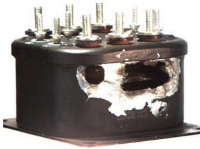
Figure 3: Relay destroyed by whisker-induced metal vapor arc
