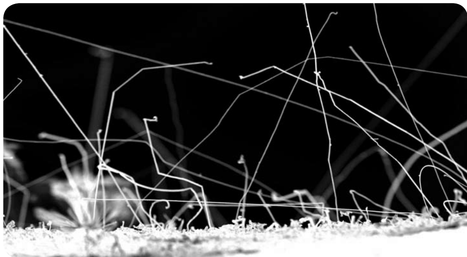
Figure 1: Zinc whiskers growing on bottom of zinc-coated raised floor tile
